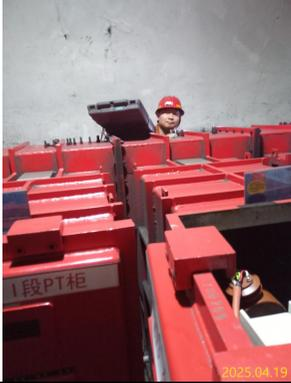
A worker in a red helmet is inspecting a red PT cabinet. The cabinet has 'I段PT柜' written on it. A timestamp '2025.04.19' is visible in the bottom right corner of the photo.                                 |
